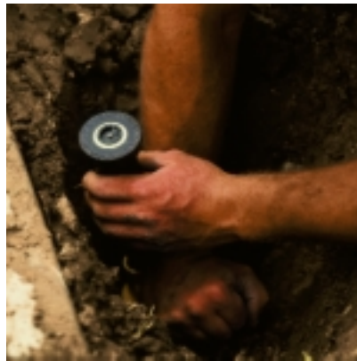
Installing the Rain Bird 1800 Series
