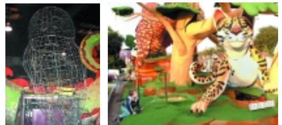
(L) Float under construction and final test run.
