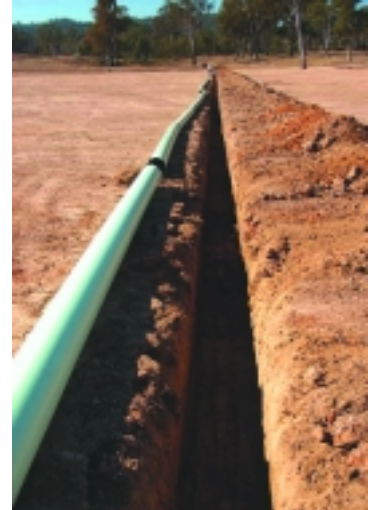
Irrigation lines are laid well before any above-ground construction begins.
