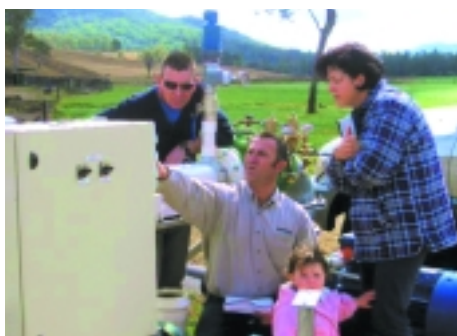
Troy Barbour, RBA (centre) and Lucas & Mandy Kennedy with the MDC control system
