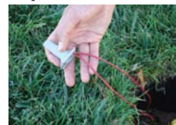
3 x 10ga and 1 x 18ga Wire Connection
