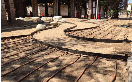
Installation of QF Dripline Header and XFS Subsurface Dripline.
