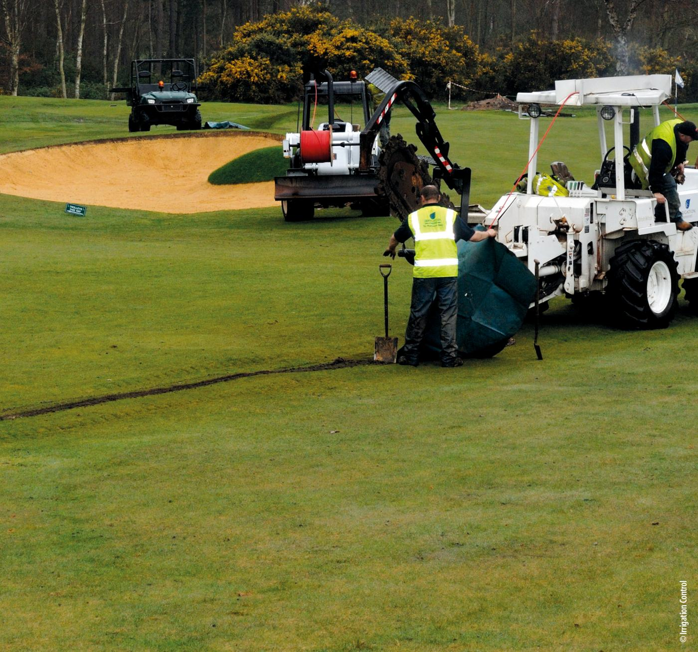
**R**enovating a golf course irrigation system is not an undertaking to be taken lightly. Whether it's a complete system renovation or a partial one, following a seven-step renovation roadmap makes the process easier and less disruptive. Some key players share their experiences to help those considering a renovation in the future...
