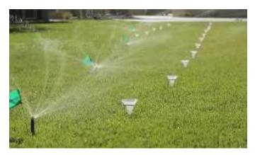
that does not receive enough water. The reason being is that inefficient systems may be programmed to run longer than what is really needed to make up for areas that don't receive enough due to improper spacing or lack of water pressure.
