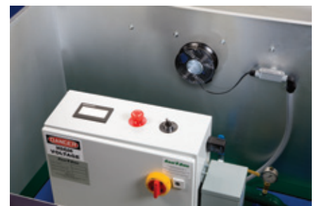
Rain Bird Low Profile Pump Station (LP) with NEMA 3R enclosure
