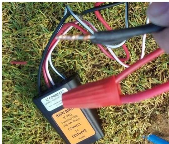
5. Add suitable protection to the splices using Rain Bird WC series wire connectors.
