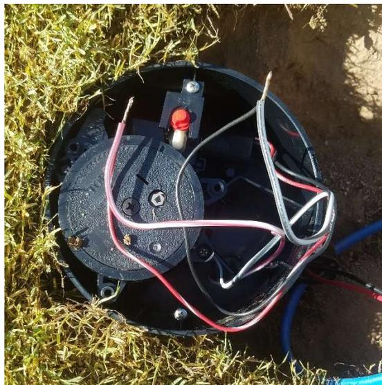
3. Add suitable protection to the splices using Rain Bird WC series wire connectors.
