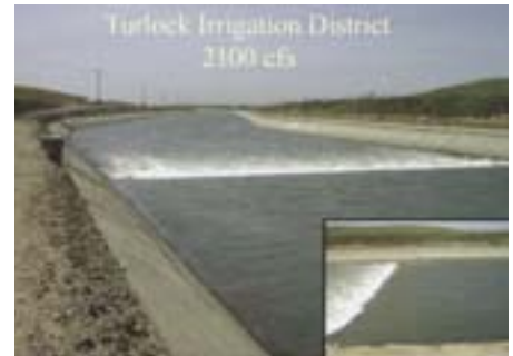
Figure 1. New Replogle Flume installed at the Turlock Irrigation District
