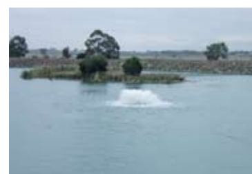
5hp High Volume industrial aerator operating at Craigieburn GC, Melbourne
