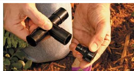
Use an Easy Fit Tee and Female Adapter, to attach a PolyFlex riser with 10-32 thread emitter to drip tubing.
