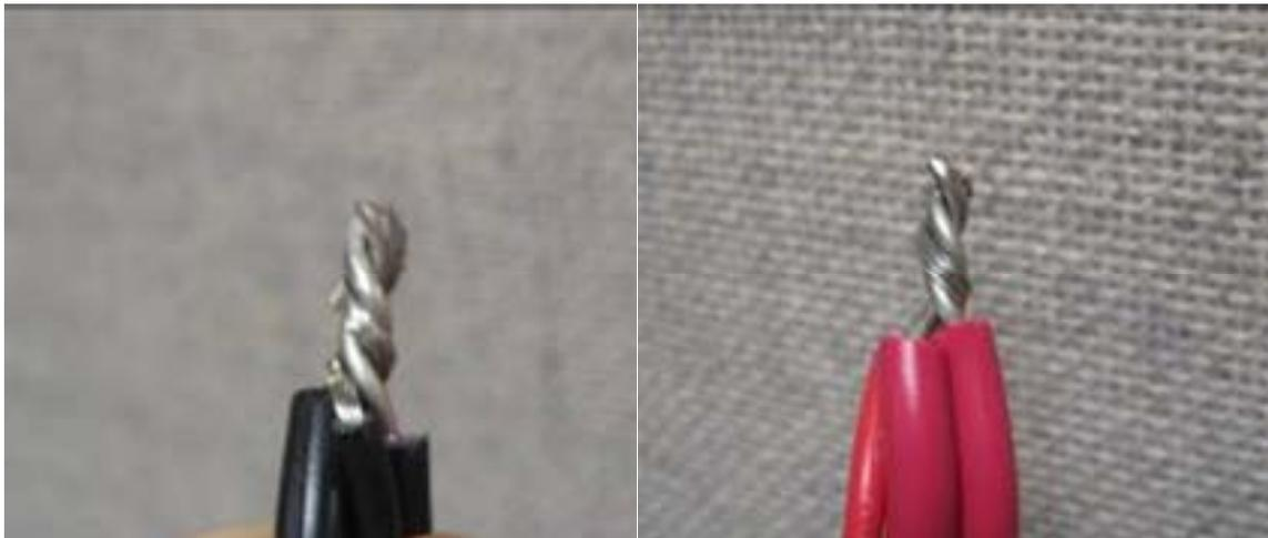
Use Rain Bird DB splice kits to ensure waterproof splices and provide strain relief. Trim the twisted bare ends of the wires to 5/8" (15.9 mm) in length before inserting in the DB splice kit. The DB splice kit has a wire length gauge on the underside of the flange to assure proper wire length.
